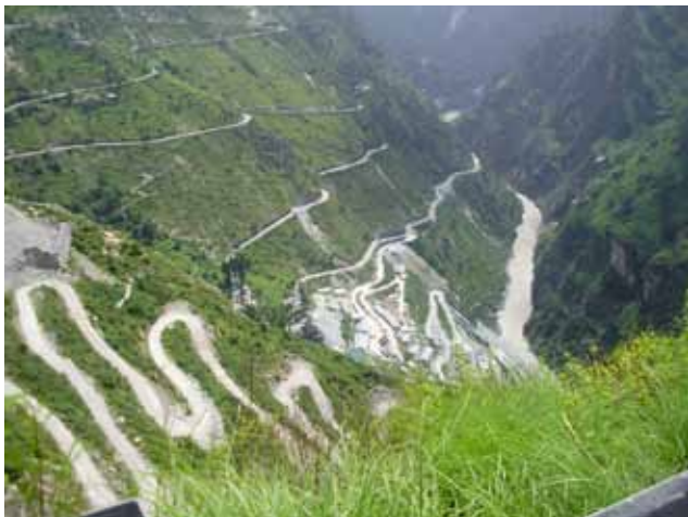
Fig. 1. The 520 MW Tapovan Vishnugad dam under construction on the Dhauliganga tributary to the Alaknanda river in Chamoli District, Uttarakhand.
