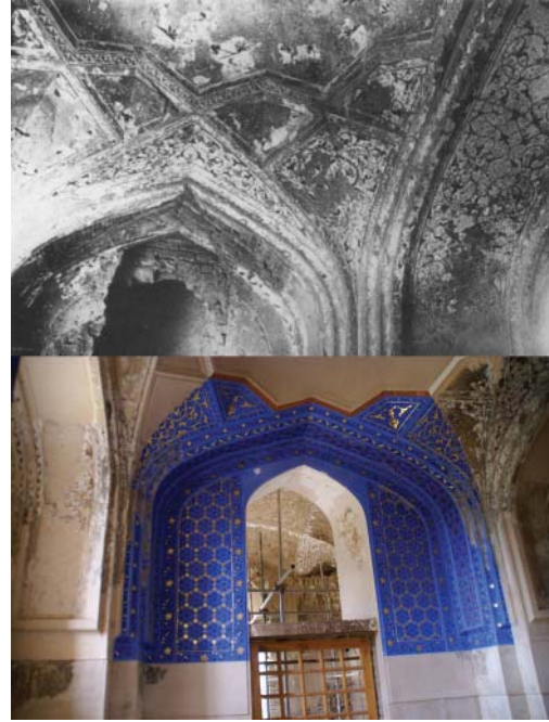
Fig. 35a, b. The Ishrat Khaneh under reconstruction, 2013, where the contrast with Pugachenkova's photo from 1963 demonstrates how much of the interior decoration is being created de novo.
