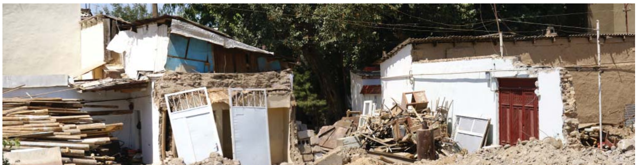
Fig. 8. The old town behind the Registan wall (composite photo 2013).
