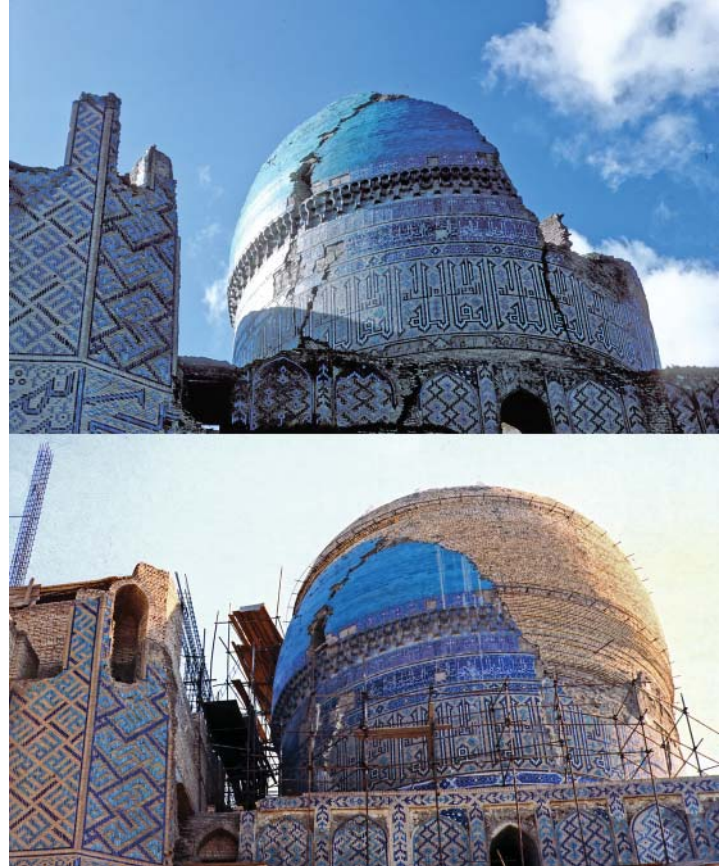
Fig. 16. The dome of the main sanctuary of the Bibi Khanum, still broken in 1969, and rebuilt but not yet tiled in 1979. (Photos © Daniel C. Waugh.)
