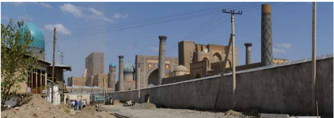
Fig. 5. Composite image showing the north side of the Registan wall, with work underway on the new road and the destruction of the adjoining houses in August 2013.
