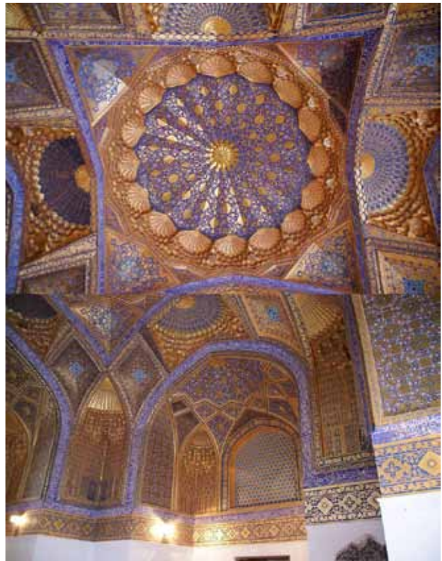
Fig. 30. The Ak Saray interior decoration after restoration, 2013.
