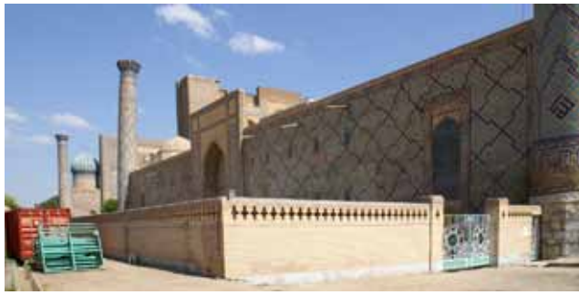
Fig. 34. The wall and gate behind the Ulugh Beg madrasa, 2013.
