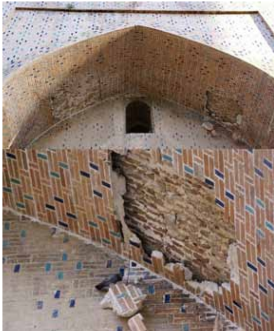
Fig. 14. The iwan arch of the southern small mosque of Bibi Khanum, with its disintegrating brickwork, 2013.
