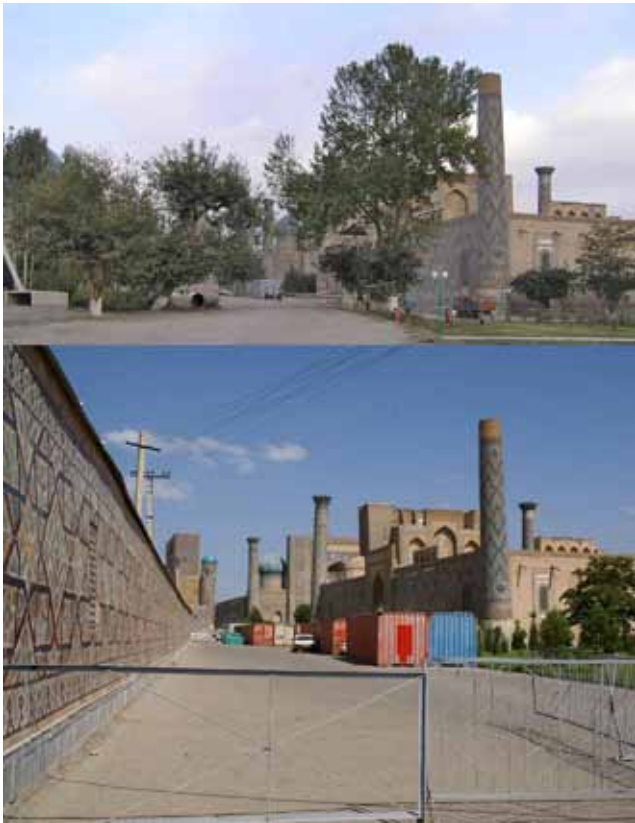
Fig. 4. View along northern side of Ullugh Beg madrasa in 2005 (photo courtesy of Gwen Bennett) and after the erection of the wall in 2013.
