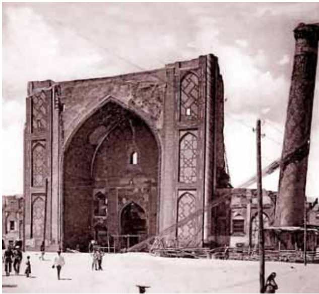
Fig. 2. The straightening of the northeastern minaret of the Ulugh Beg madrasa in 1932. (Source: < http://mytashkent.uz/2012/12/09/k-80-letiyu-vypryamleniya-minareta-vladimir-grigorevich-shukhov/ >.)
