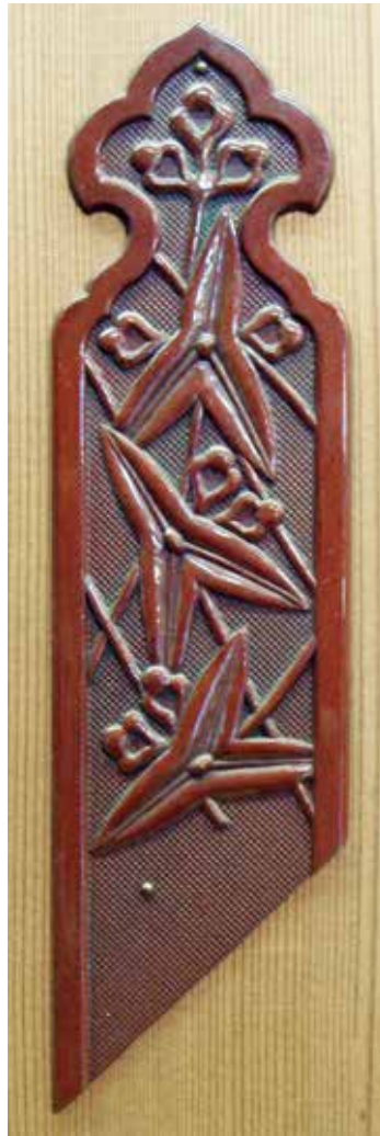
Fig. 4. Suaka or Akagane is an artificially red/orange patinated alloy, containing 1-2% of zinc and/or lead. Modern architectural fitting, Morimoto Kazari, Kyoto. (Photo by author)
