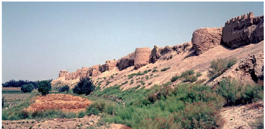
Fig. 4. Balkh. The Timurid walls of the Bala Hissar. Photograph copyright © 1970 Ruth Harold.
