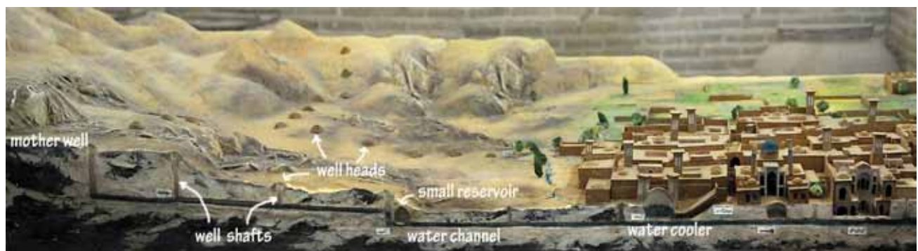
Fig. 2. Model of qanat supplying water to the city of Yazd, Iran. Photo (composite image) © 2010 Daniel C. Waugh taken at the Water Museum in Yazd, Iran.
