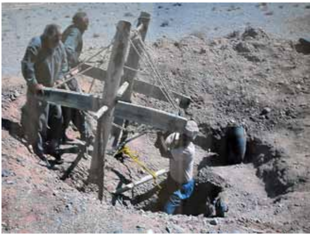
Fig. 3. Workers digging a qanat. Photo © 2010 Daniel C. Waugh, from a photo in the Water Museum, Yazd.
